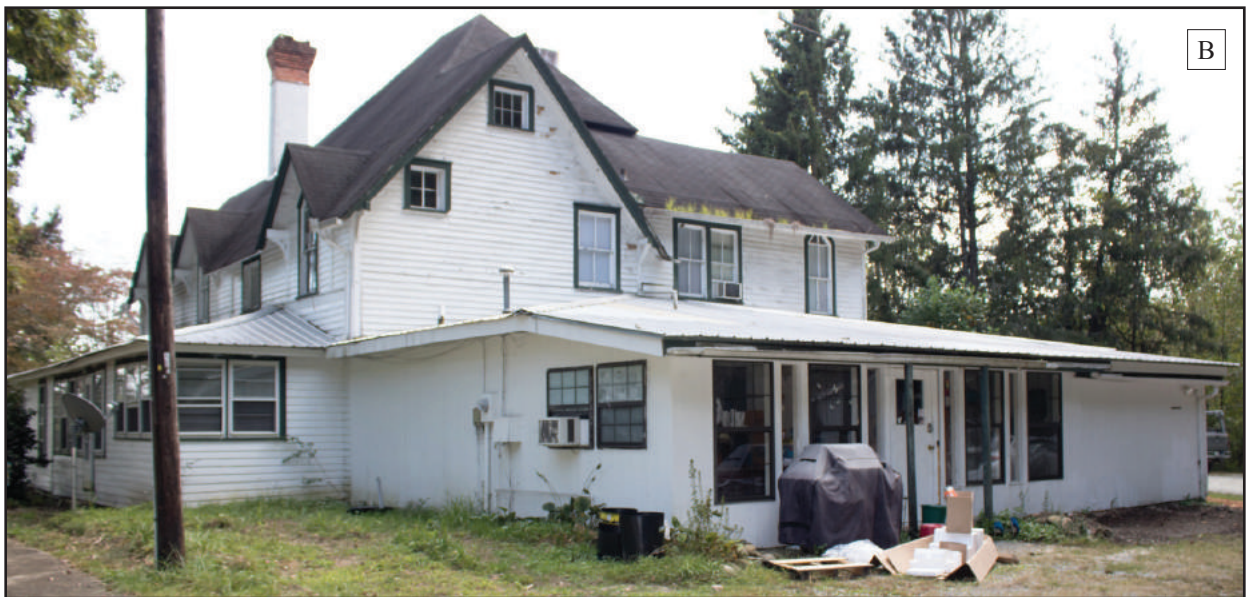
Figure 6.6. Robert E. Patton House Additions
