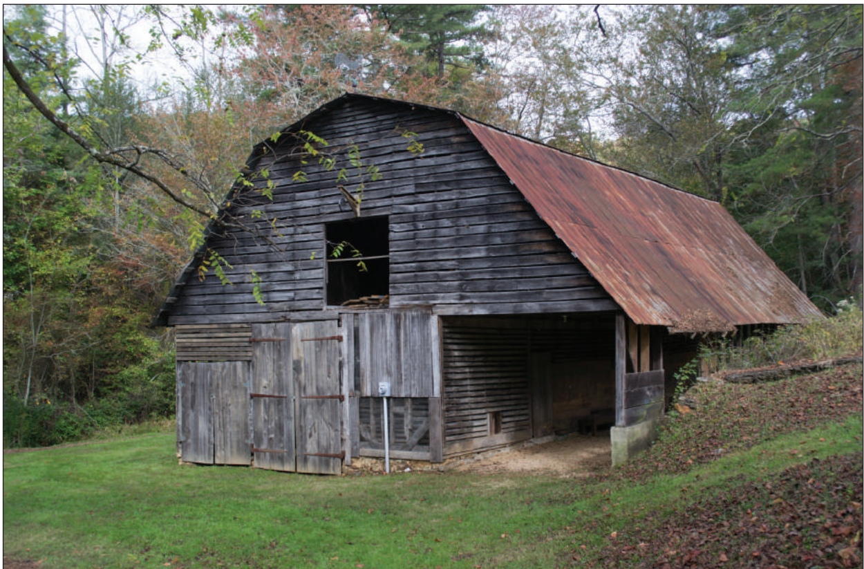
Figure 3.5. Barn, Looking North
