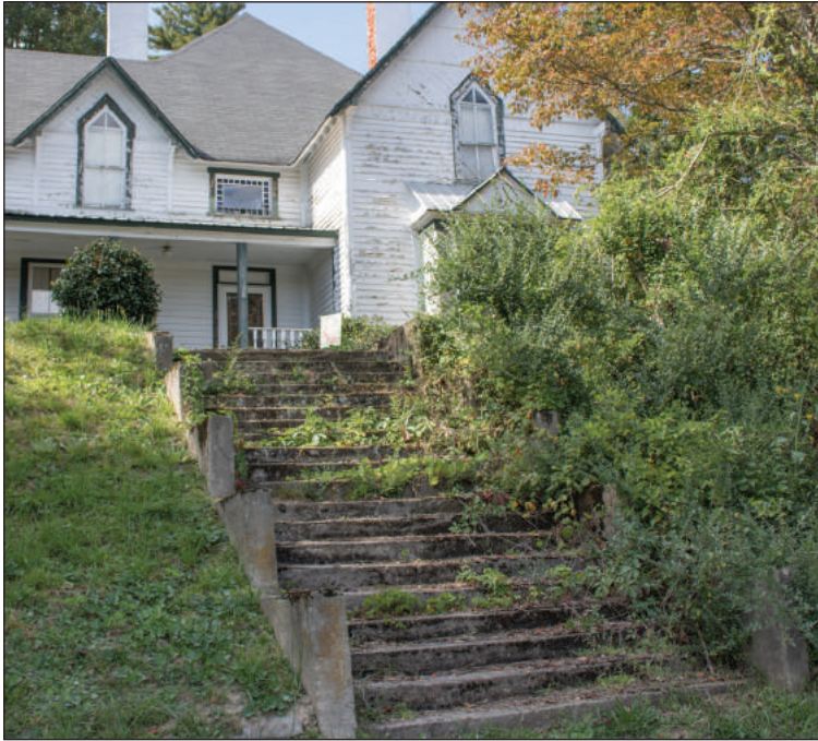
Figure 6.2. Robert E. Patton House, Concrete Stairs, Looking Northwest
