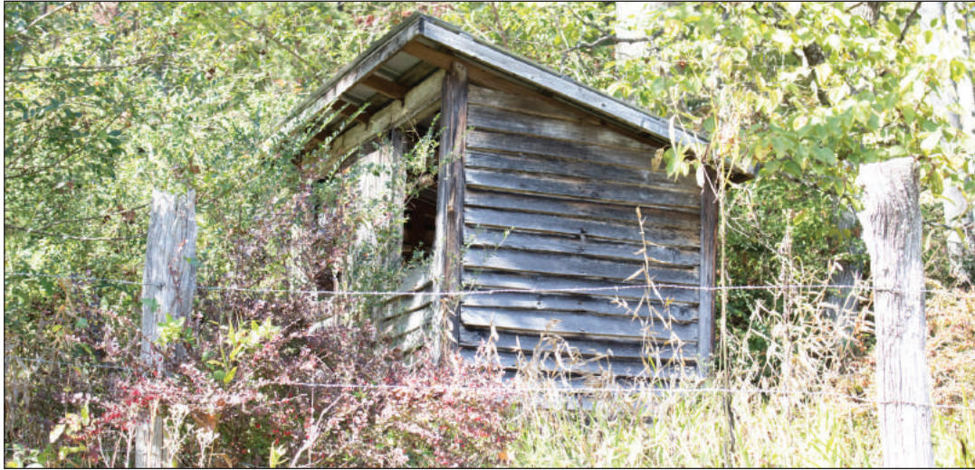
Figure 7.6. Chicken House, Looking North
