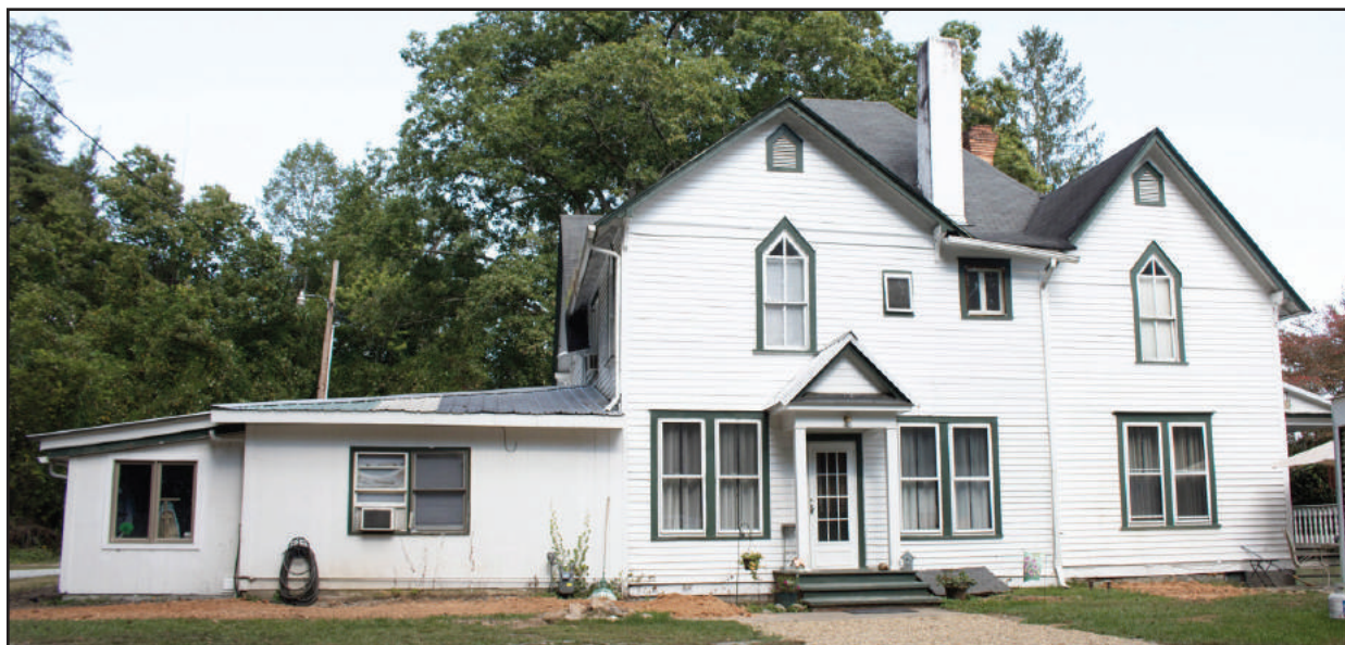
Figure 6.7. Southwest Side, Looking Northeast
