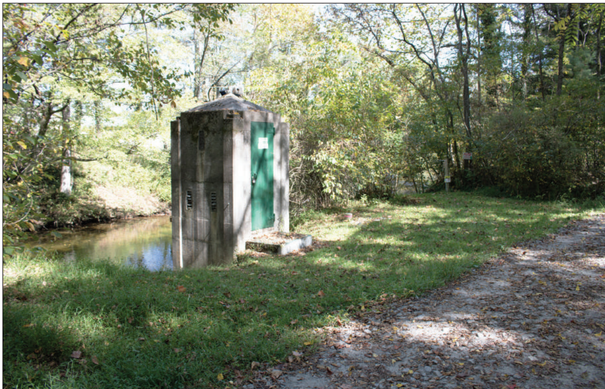
Figure 4.2. Davidson River Gaging Station, Looking East
