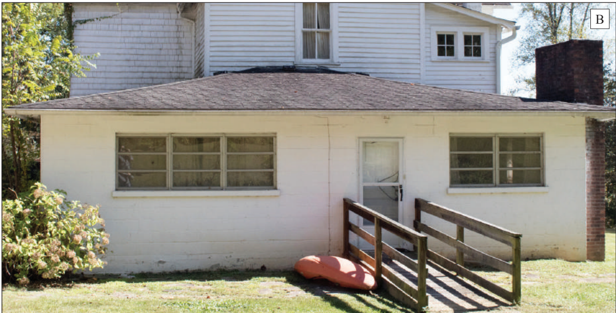
Figure 7.5. Rear of the House
