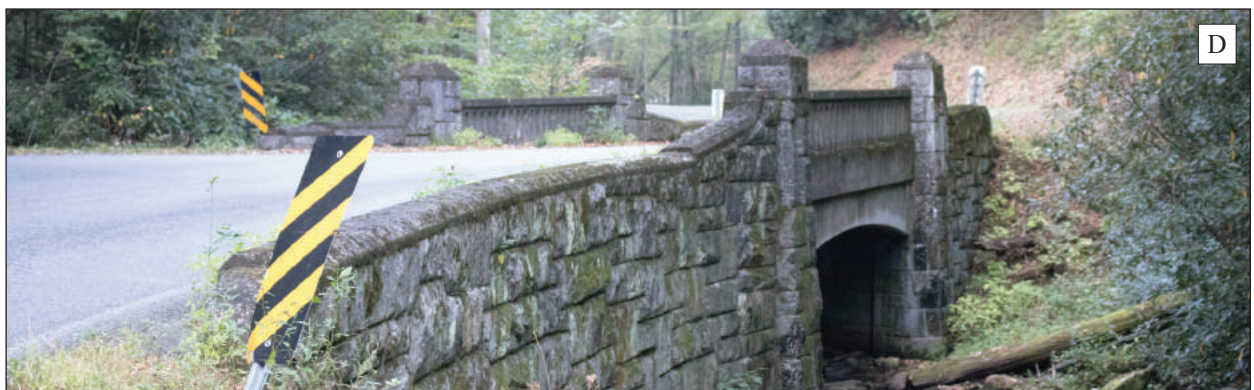
Figure 5.7. Pisgah National Forest Bridges (TV0482)
