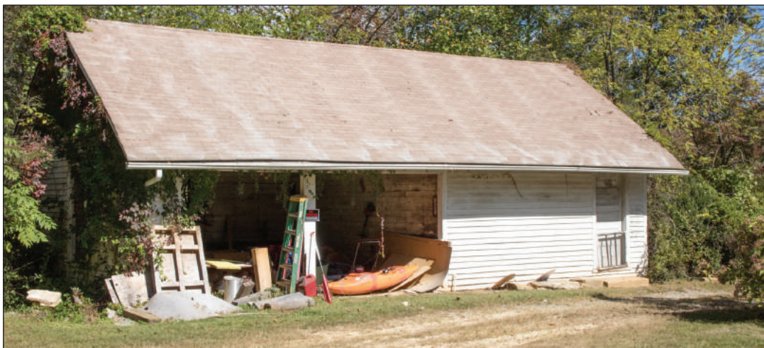
Figure 7.7. Garage, Looking East
