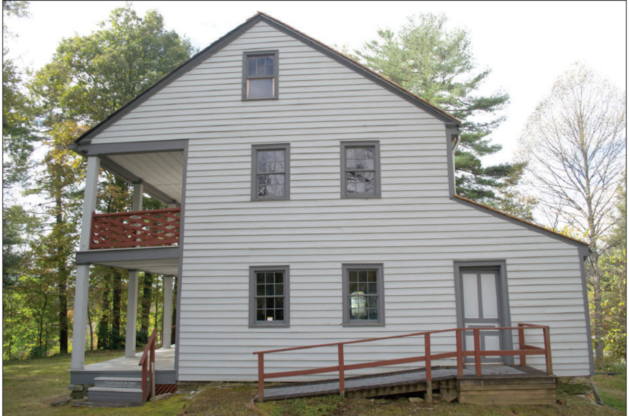
Figure 3.3. Northeast Elevation, Looking Southwest
