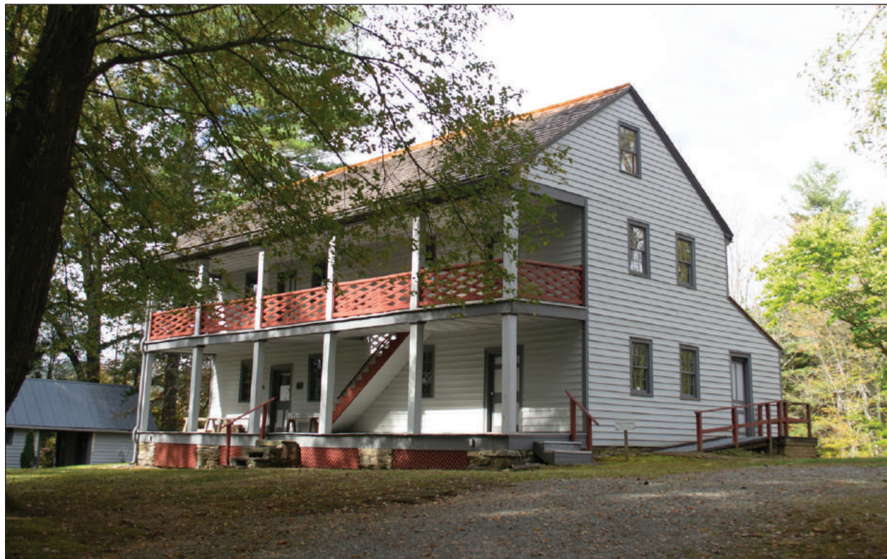
Figure 3.2. William Deaver House, Looking West
